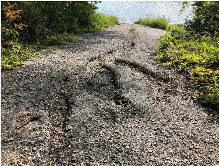
Photos 25-26: Signs of Erosion on boat launch area (left), and Mount Hope Road drainage leading to area (right)
