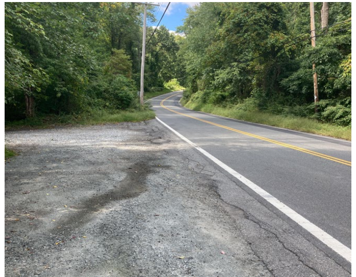
Photos 25-26: Signs of Erosion on boat launch area (left), and Mount Hope Road drainage leading to area (right)
