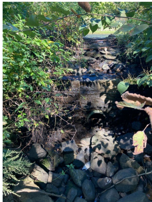
Photos 35-36: Current conditions of side rock-lined swale and Outlet structure of retention pond, showing outlet area blocked
