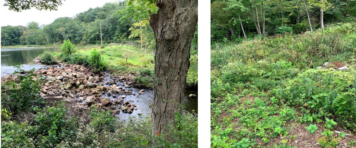
Photos 21-22: Hiberina brook outflow along Lake Ames impoundment (left) & vegetation along backside of the impoundment
